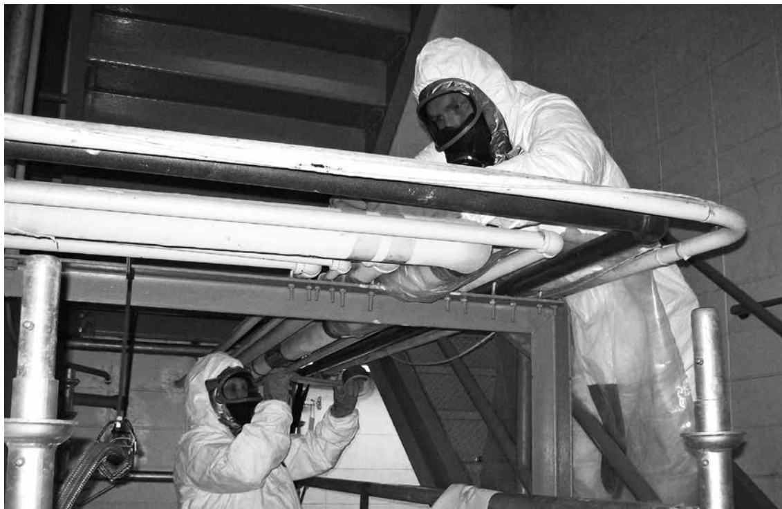
“Asbestiving/sanering. Kilde Wikimedia Commons”
